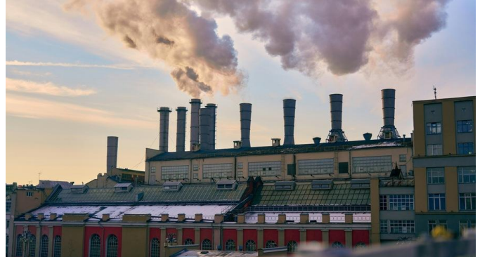
Stacks, ducts, boilers & process control
