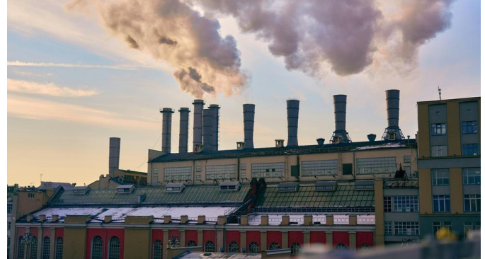
Stacks, ducts, boilers & process control
